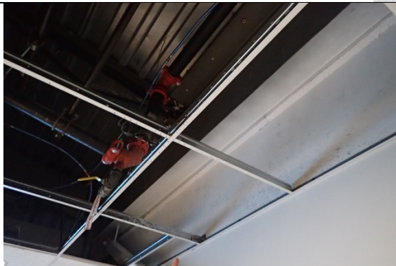
Fig. 2.1a. Replaced sprinkler fittings. Rigid insulation added between wall and wide flange beam.
