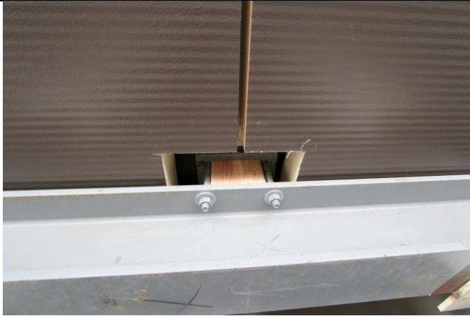
Figure -1.1a. Gap at pile cap as seen during conduction on April 3, 2014
