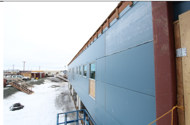
Fig. 2.1e. Eave condition on north end of building, as seen on April 3, 2014 Construction Observation Site Visit.
