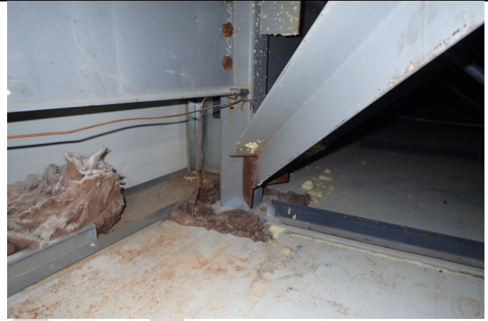
Figure -1.1b. Batt insulation added to fill gaps at pile cap and soffit
