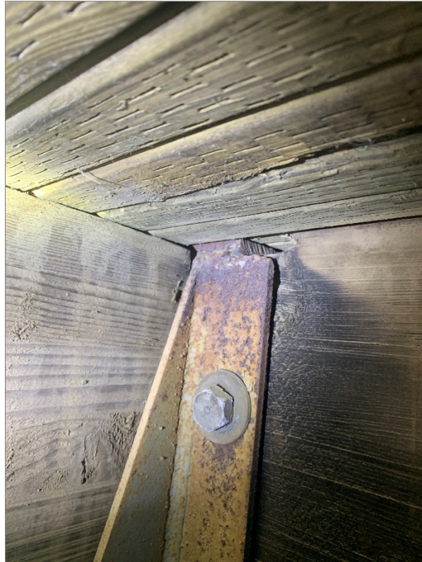
Figure: 3 – Subfloor and floor joist
