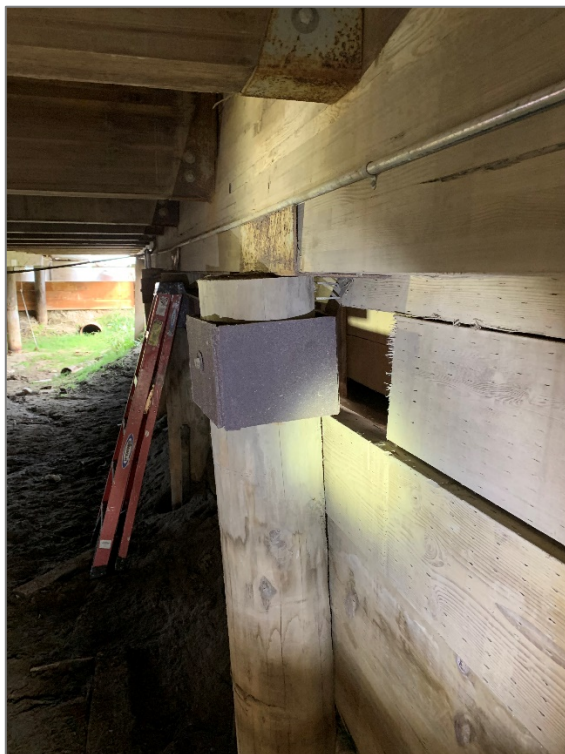
Figure: 5 – Wood piling and floor joist
