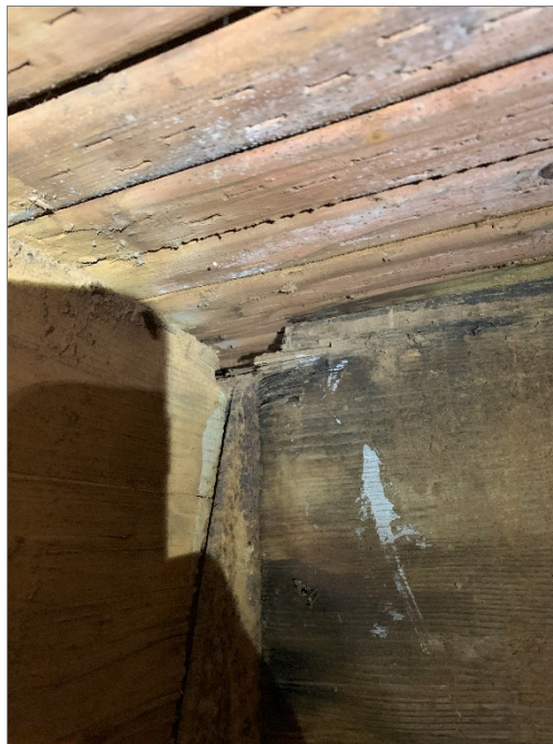
Figure: 2 – Subfloor and floor joist
