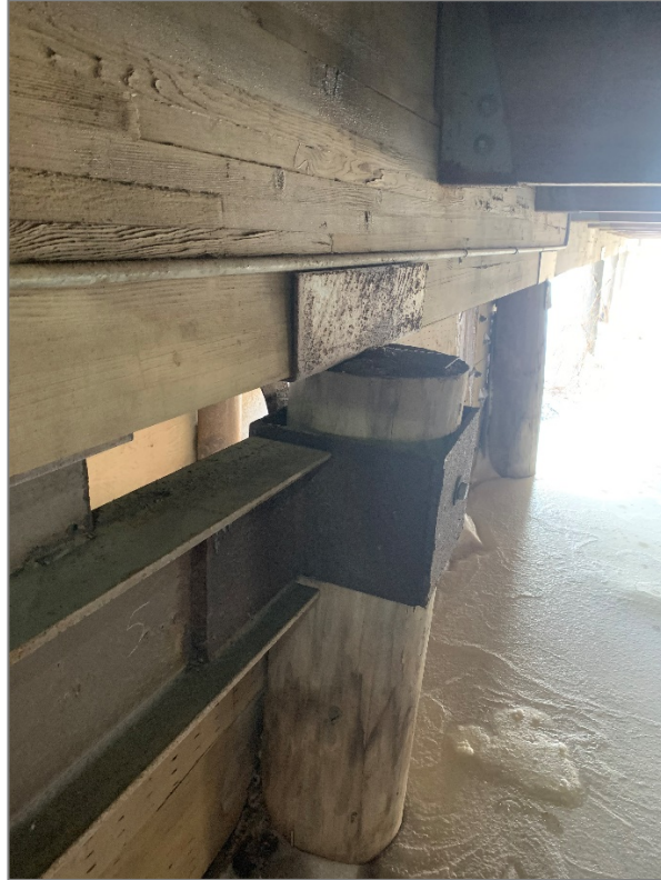
Figure: 11 – Wood piling and floor joist
