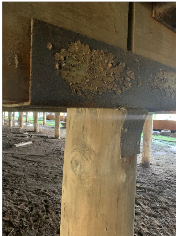
Figure: 4 – Wood piling and floor joist
