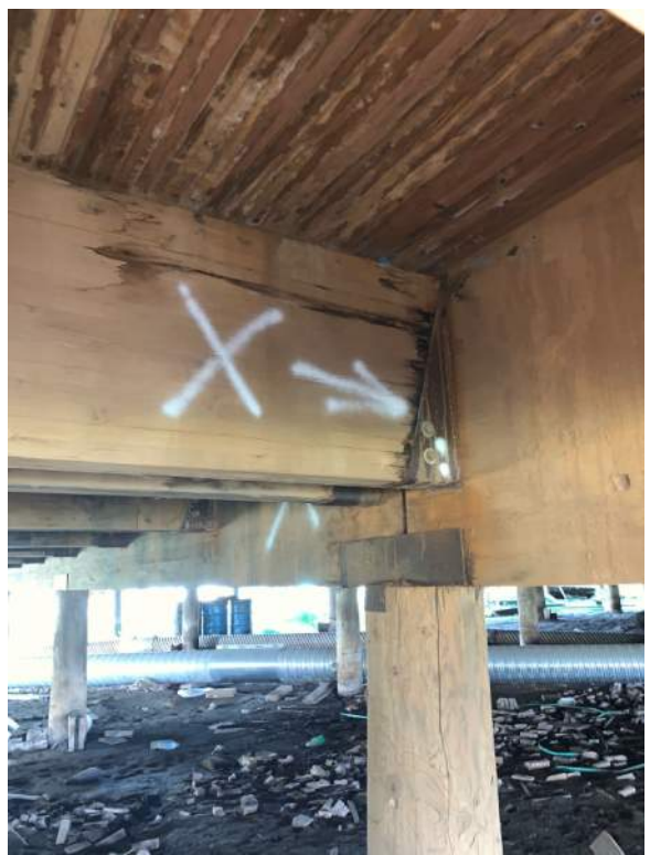
Photo 4 – Beam and Hanger Markings
