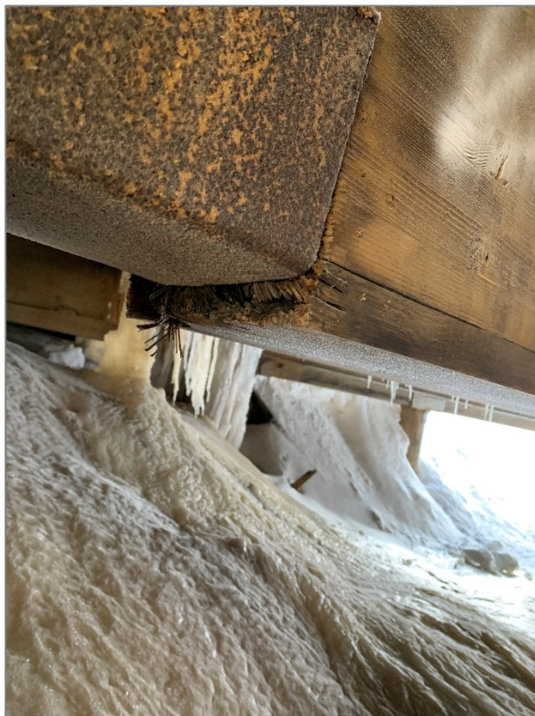
Figure: 9 – Floor joist
