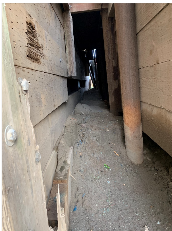
Figure: 6 – Subfloor access point
