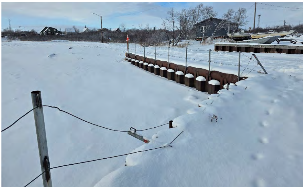
Photo 12: 30" pipe, Z-pile wall cap at DS end of 1st Ave Bulkhead at the US extent of the Float Plane Area. Pipe replaced original timber wall cap, PBL STA 69+00, 3 November 2025
