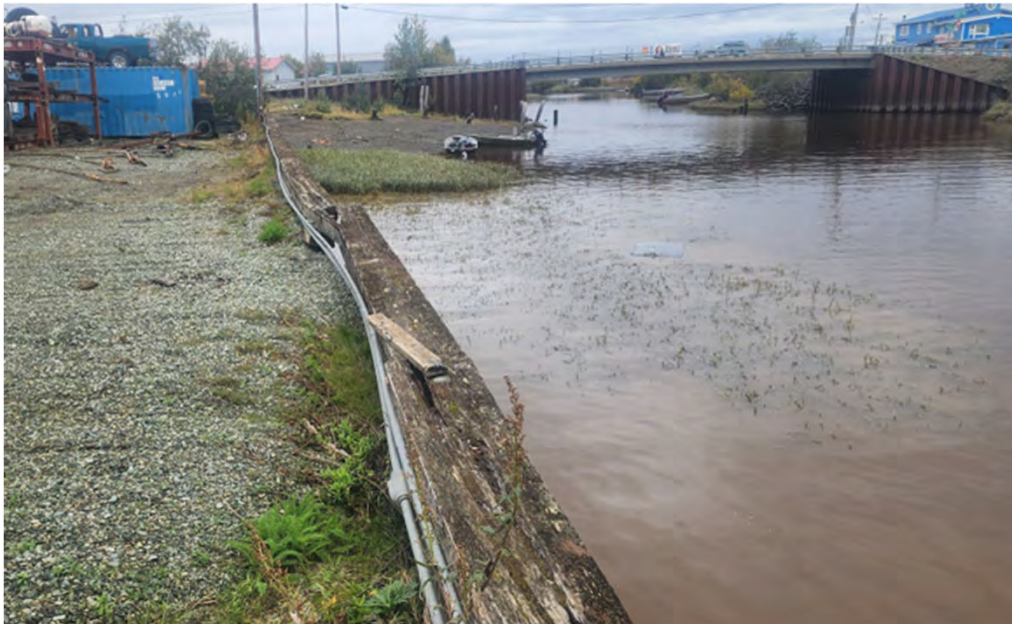
Photo 29: Failing wooden retaining wall and railing failing on downstream side (relative to the Kuskokwim River) of Brown's Slough, Approx. PBL STA 94+00
