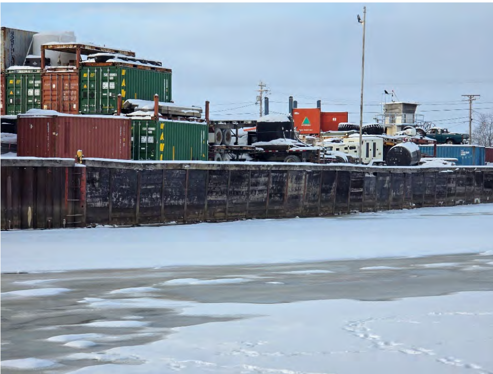
Photo 30: Failing retaining wall on downstream side (relative to the Kuskokwim River) of Brown's Slough, Approx. SCL STA 10+00
