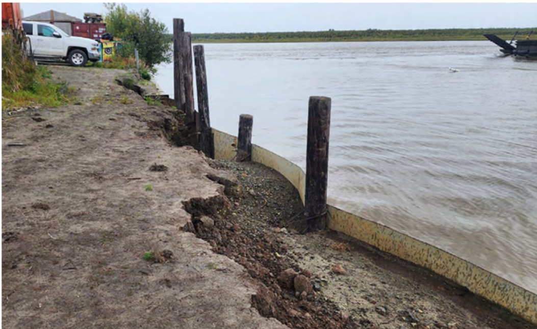
Photo 32: Failing sheet pile on upstream side (relative to the Kuskokwim River) of Brown's Slough, Approx. SCL STA 10+00
