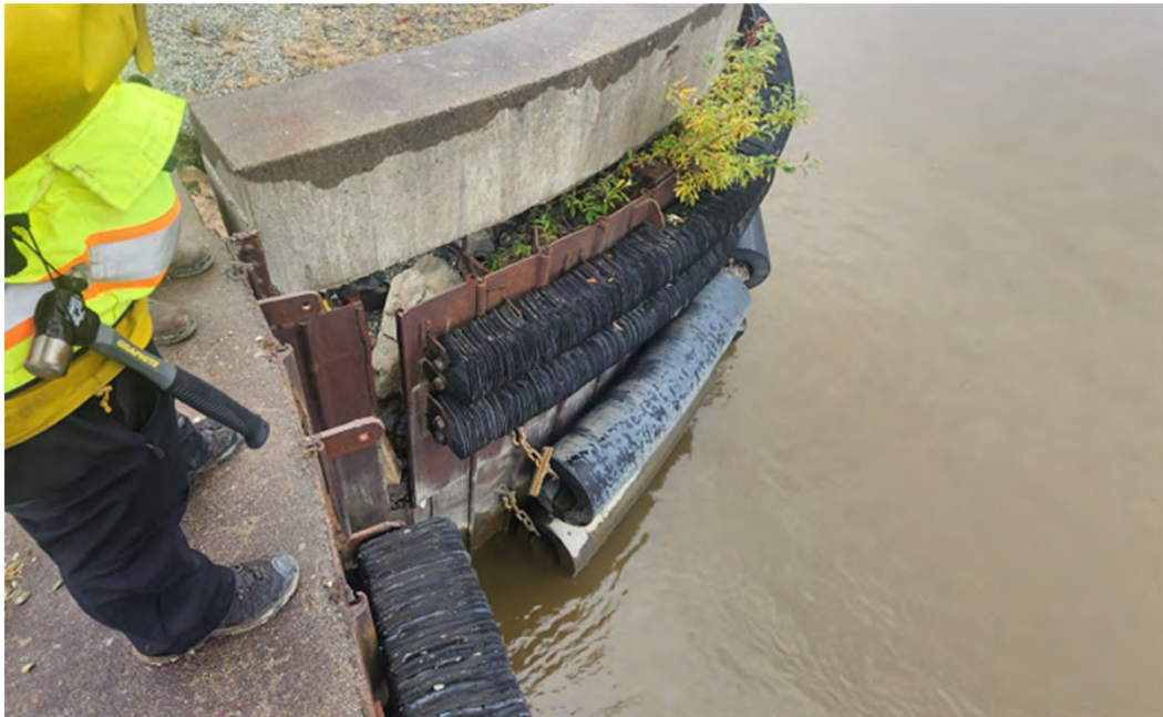
Photo 25: Failed sheet pile interlocks at US end of City Dock, photo taken 4 September 2024 at 1543, Approx. PBL STA 93+40
