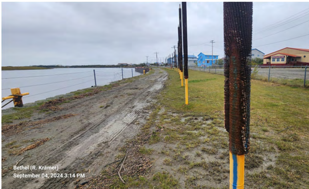
Photo 16: Rusted condition of cooling fins on thermotubes (also known as thermosiphons), Approx. PBL STA 77+00
