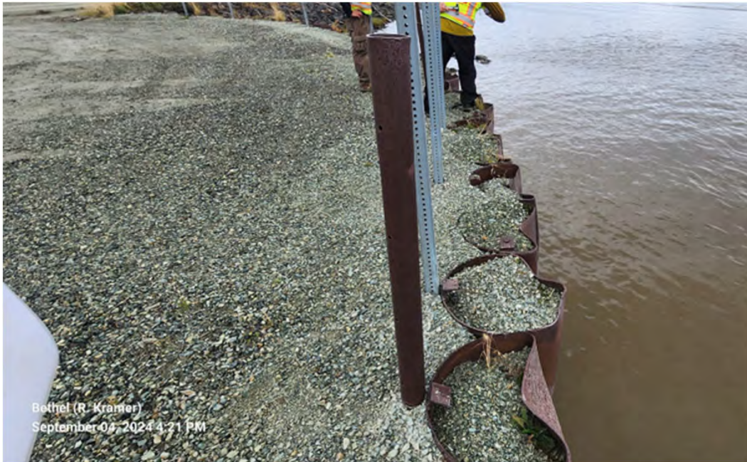
Photo 21: Gravel surfacing appears to have helped block surface drainage path between filter fabric and washout protection angles noted in past reports, Approx. SCL STA 20+50
