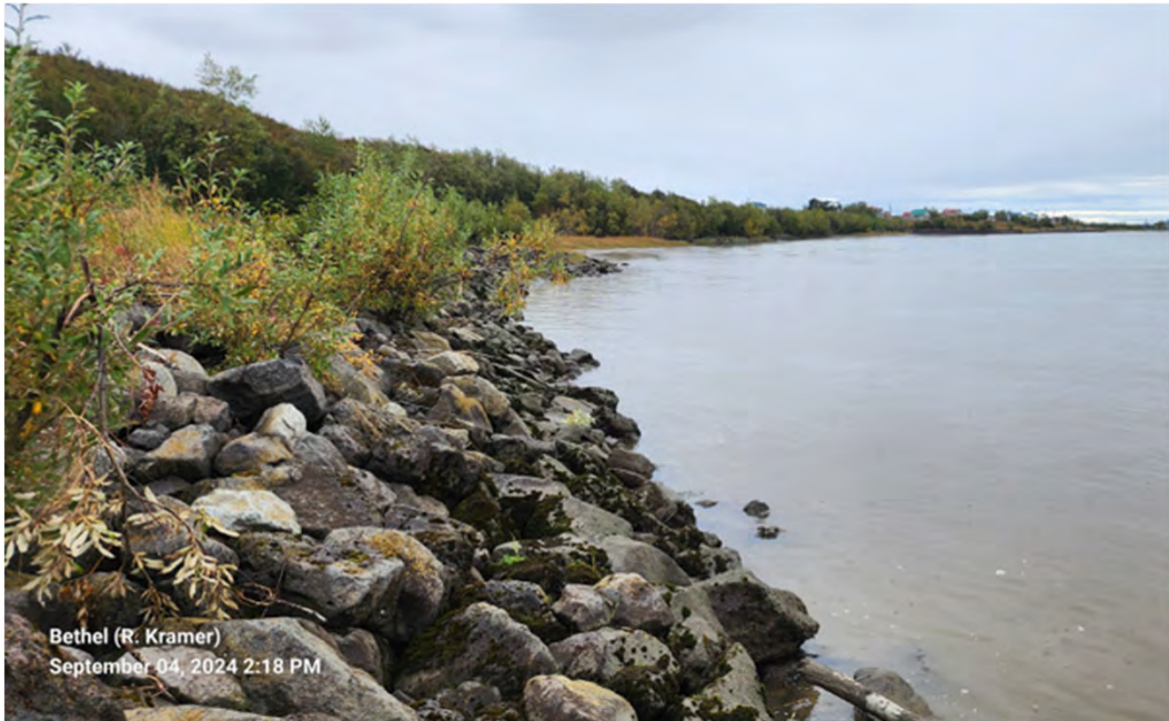
Photo 7: Typical conditions along the rock revetment US from Beach 2 where tree cutting has been completed, Approx. PBL STA 32+00
