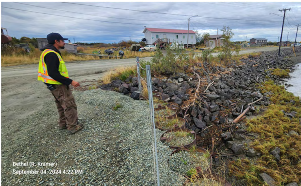
Photo 22: Riprap at US end of East Bulkhead, SCL STA 21+50
