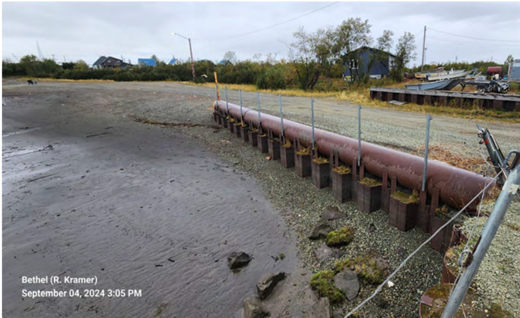
Photo 11: 30" pipe, Z-pile wall cap at DS end of 1st Ave Bulkhead at the US extent of the Float Plane Area. Pipe replaced original timber wall cap, PBL STA 69+00, 3 November 2025
