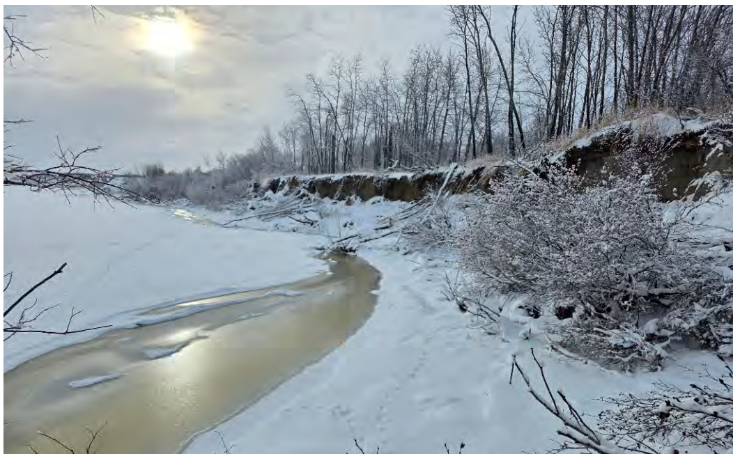
Photo 2: Snow-covered area DS from end of revetment, PBL STA 11+74, 3 November 2025
