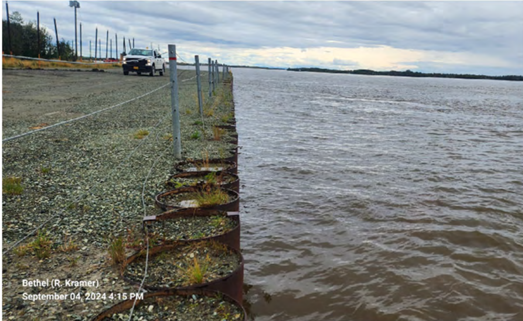
Photo 19: East Bulkhead looking US at area with exposed “B” rock, Approx. SCL STA 13+50
