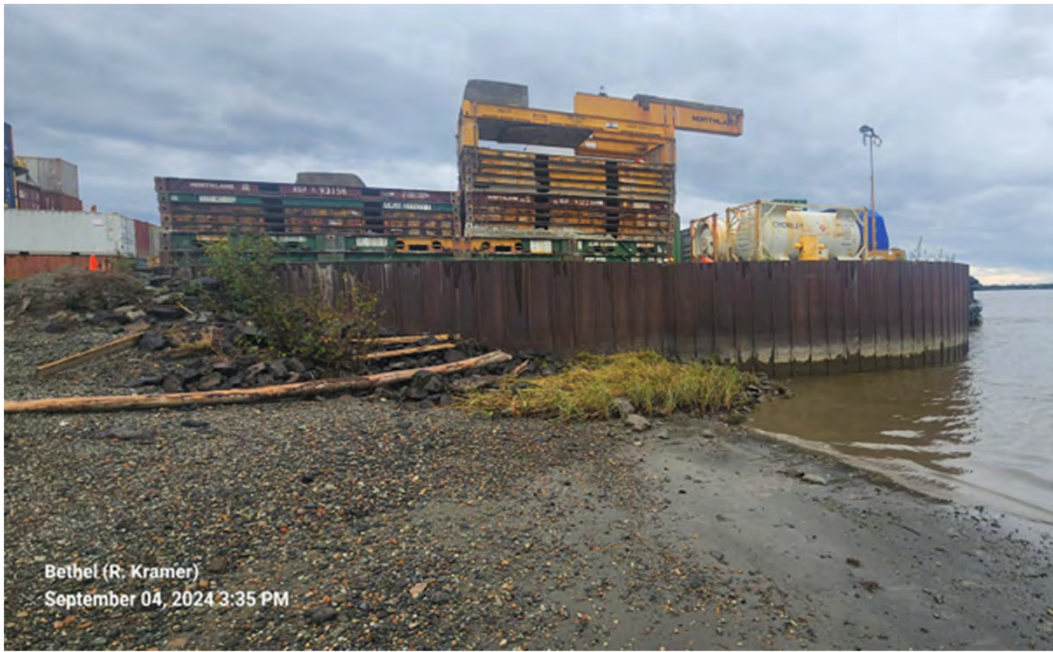
Photo 17: DS extent of City Dock, PBL STA 90+50
