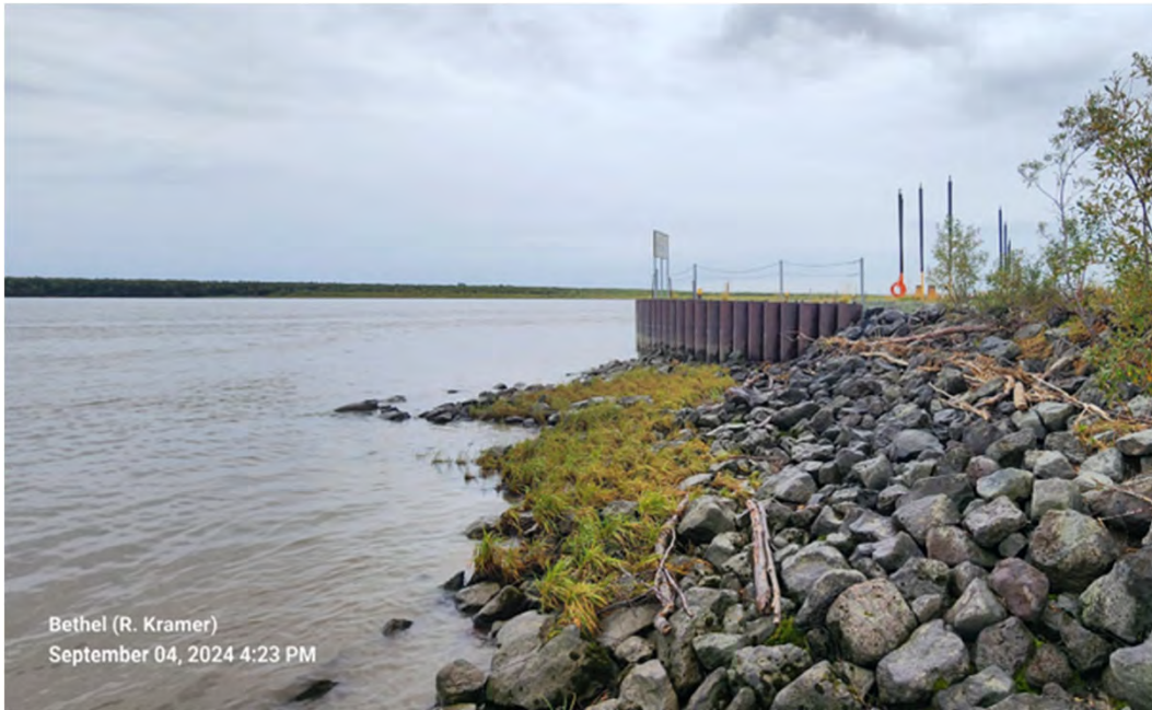
Photo 23: US end of East Bulkhead facing DS, SCL STA 21+51
