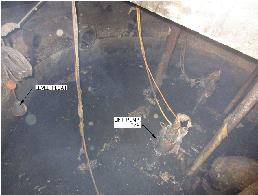
4 WET WELL INTERIOR E-603 SCALE: NTS
