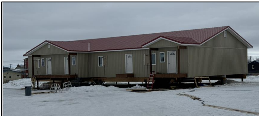
Professional Housing Building
