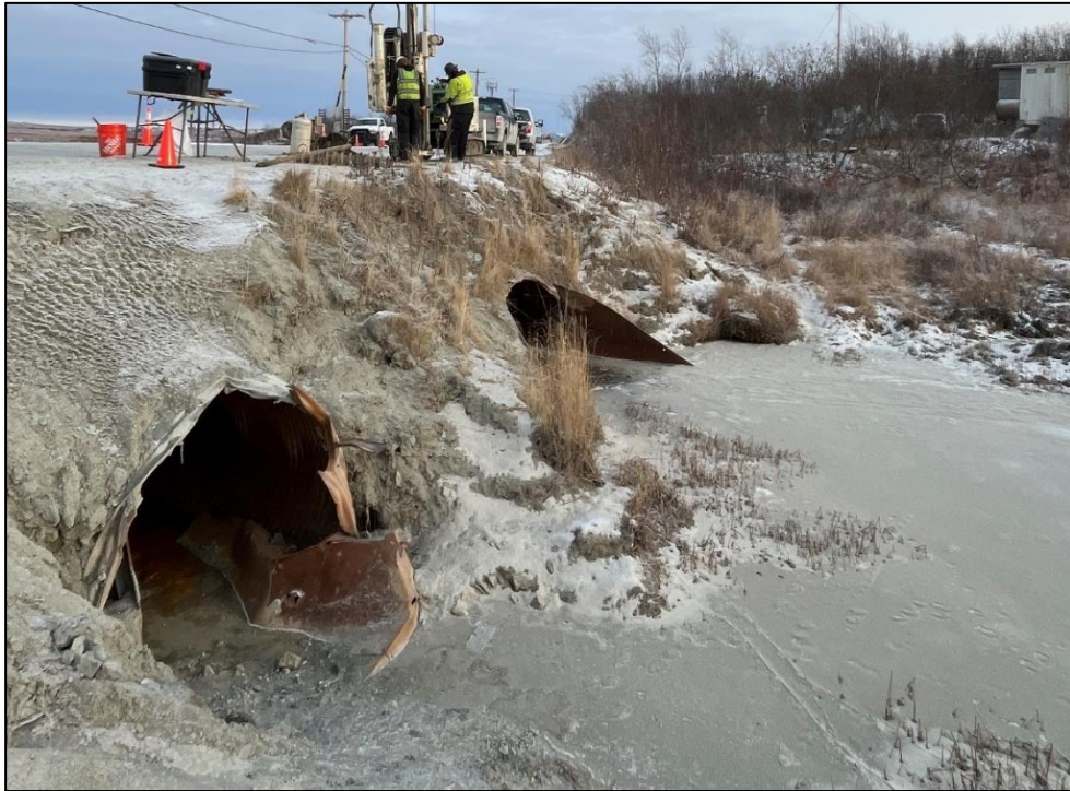
Figure 1: Site 1 culvert crossing viewed northeast.
