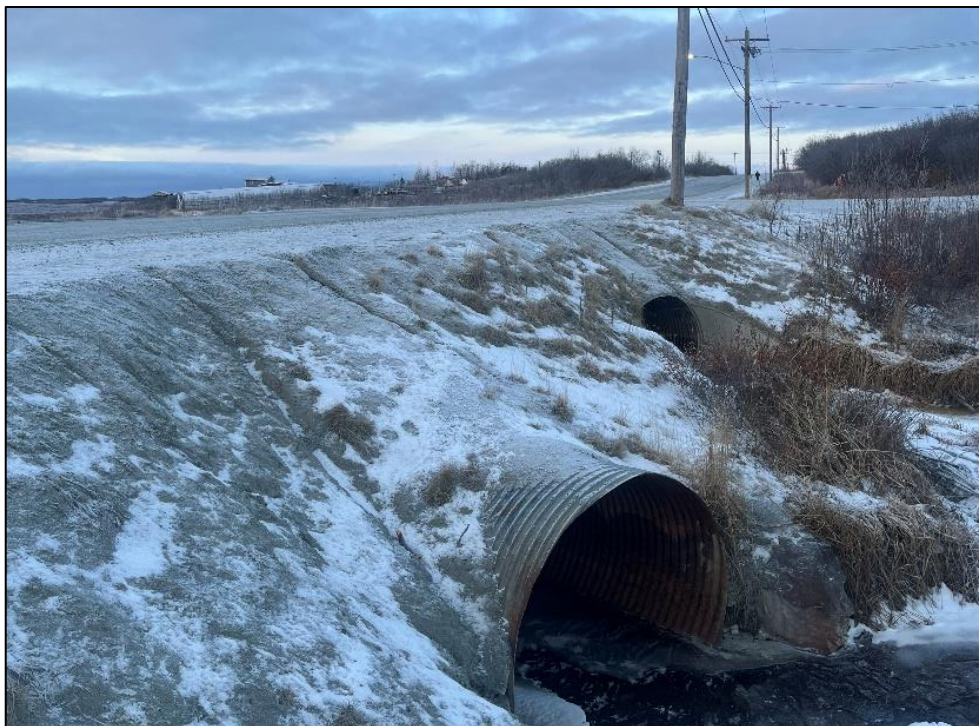
Figure 2: Site 2 culvert crossing viewed southwest.
