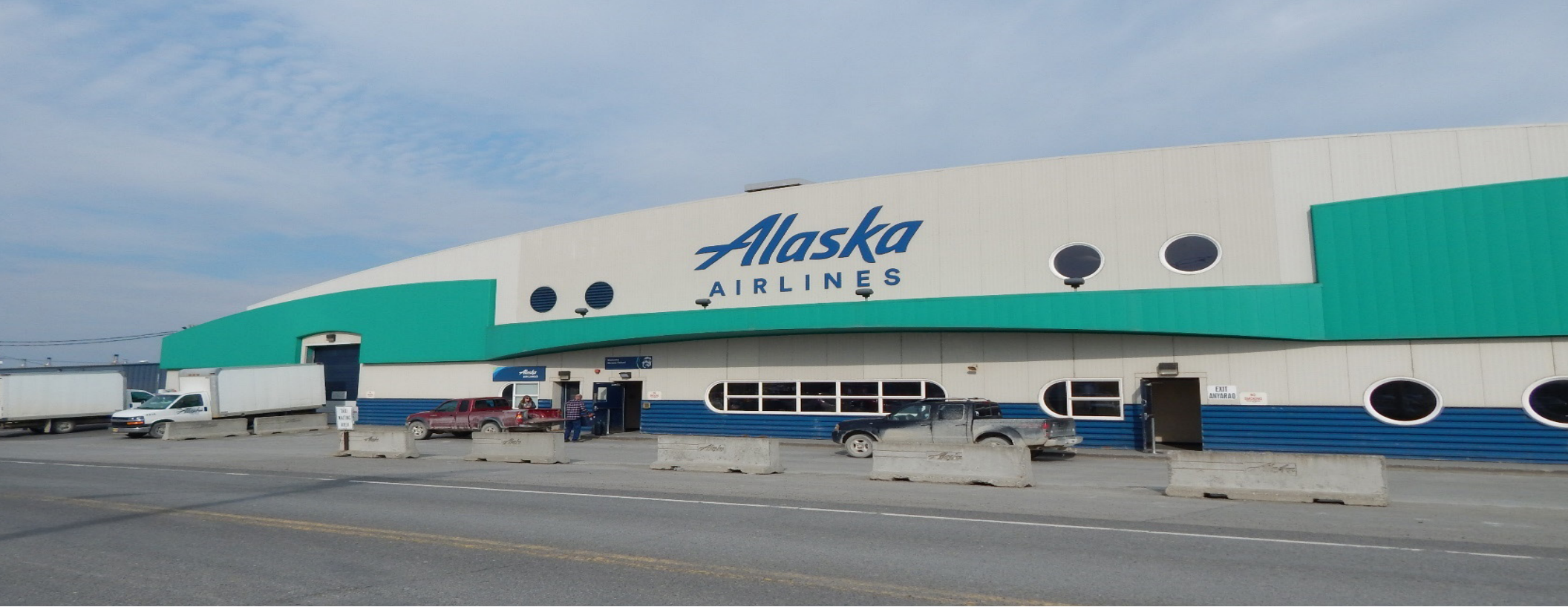
Passenger loading area in front of the Alaska Airlines terminal at the Bethel Airport.
