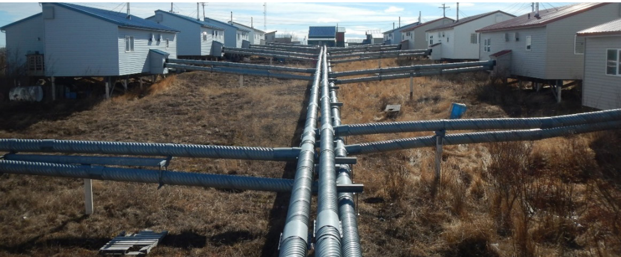
Water and sewer pipes serving homes in the Bethel Heights neighborhood.
