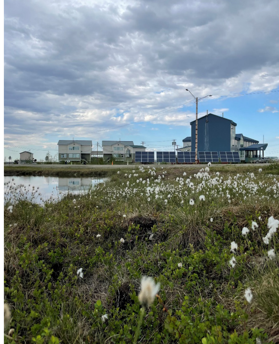
A solar array near the Fitness Center in Bethel.
