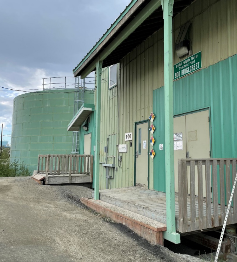
Bethel Heights water treatment plant.
