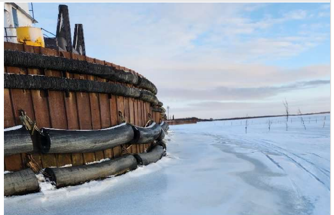
Start of fendering at closed cell, CC4
