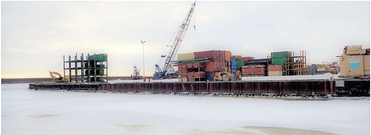
Photo 2: East Wall – Sheet Pile Segment
