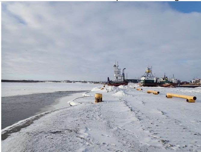
Top of dock face
