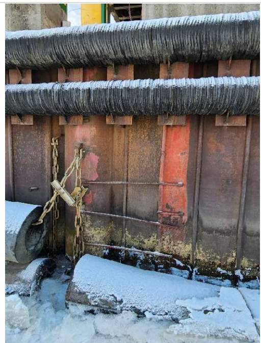
Safety ladder at soldier pile S37
