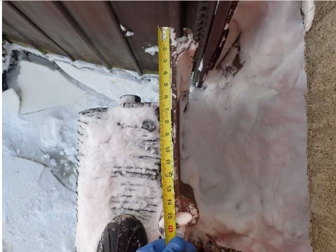
Overall length of PS28 sheet pile at east wing wall
