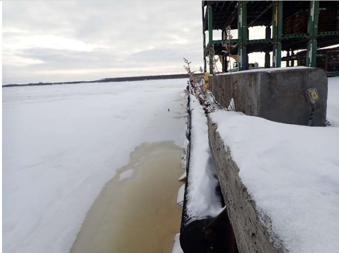
Fendering and concrete curb along east sheet pile wall
