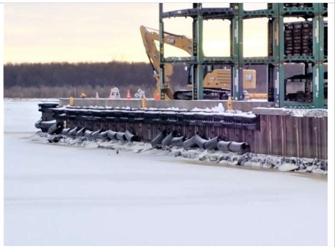
Fendering on east sheet pile wall
