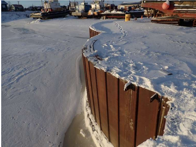
Top of west wing wall
