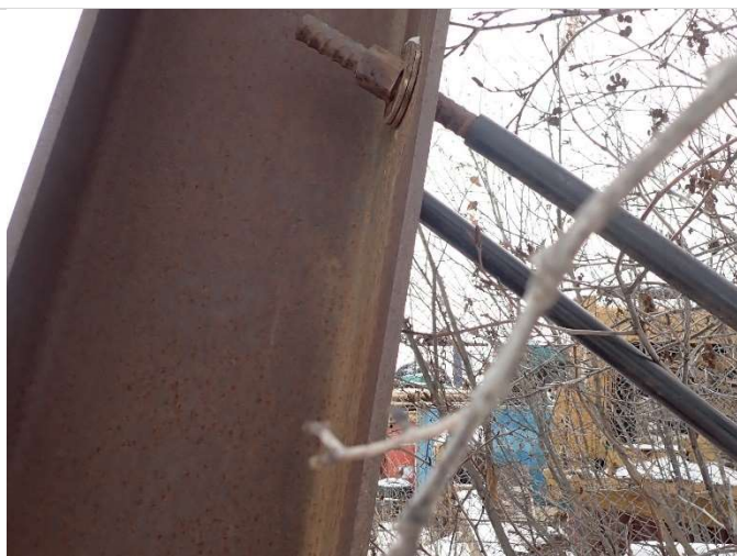
Intact HP tiebacks
