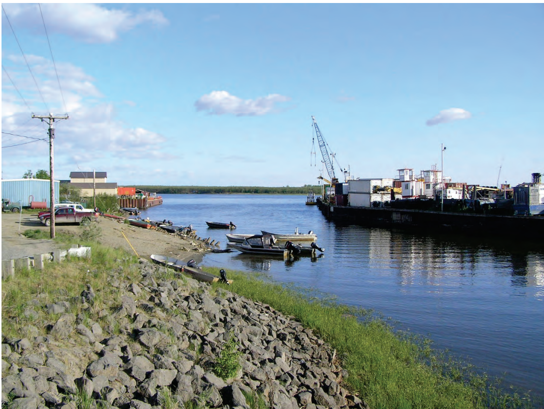
Bethel Bank Stabilization along Brown's Slough, June 2007
