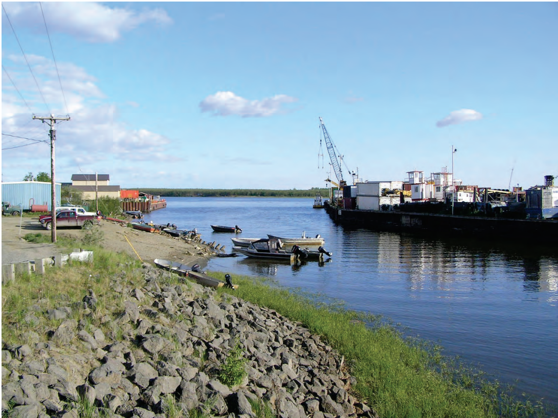
Bethel Bank Stabilization along Brown's Slough, June 2007
