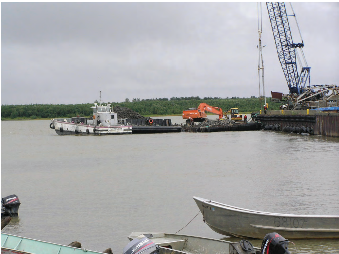
Placement of riprap, August 2007
