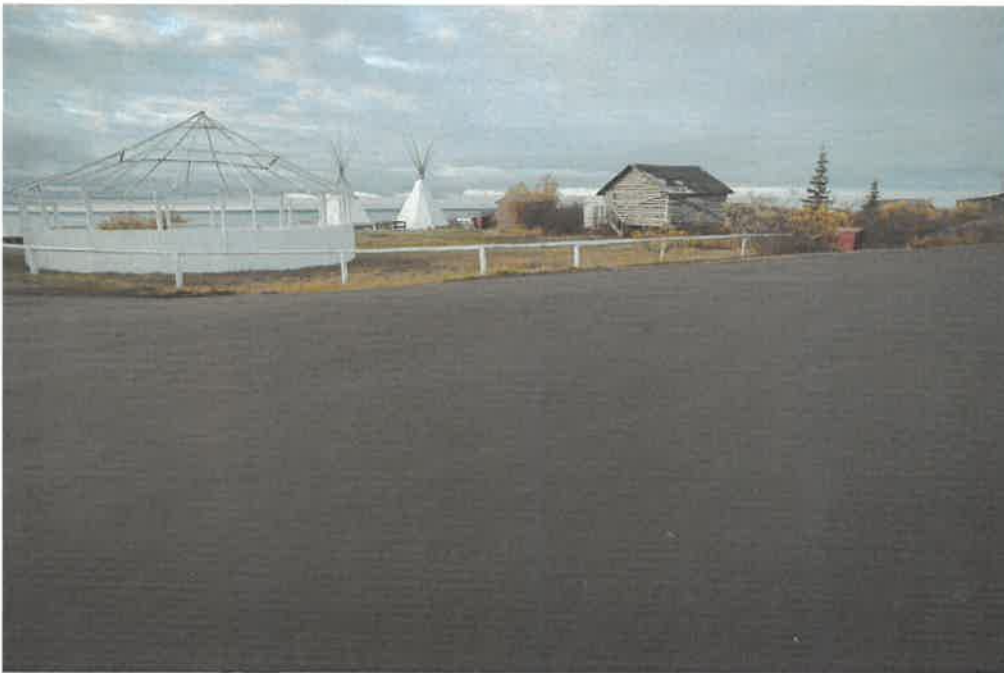
Pavement like EK35 road surface
