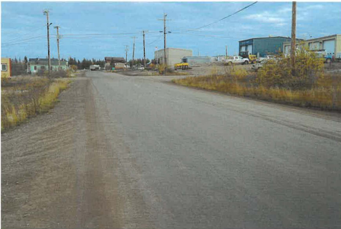
Tightly bound treated road surface
