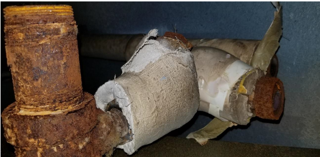
Photo 4: This photo shows a “hard elbow” on the heating unit. This material was found to be non-ACM.
