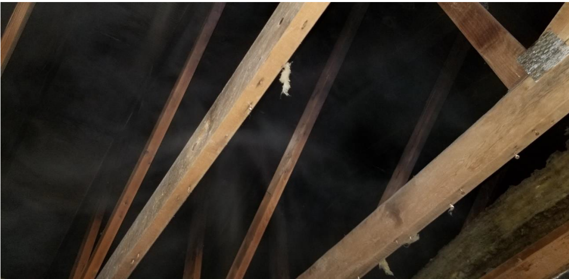
Photo 2: This photo shows the interior roof construction. It consists entirely of wood and metal on the inside.
