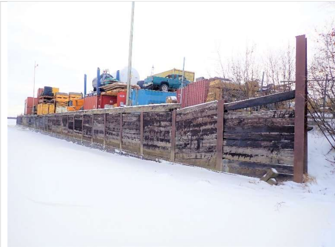
Pile jacking at north end of the timber wall
