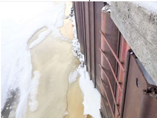
Safety ladder on east sheet pile wall
