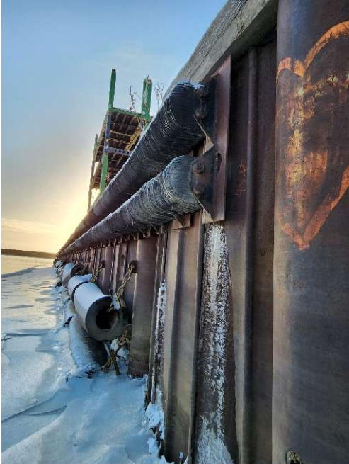
Start of east wall fendering
