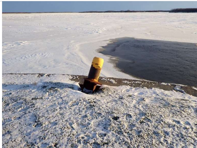
Damaged 10" dia bollard at SE corner of dock (closed cell #1)
