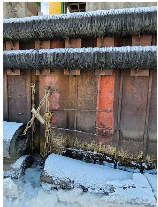
Safety ladder at soldier pile S37
