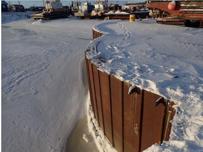
Top of west wing wall
