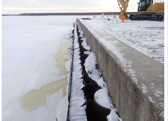
Concrete curb and fendering along east sheet pile wall
