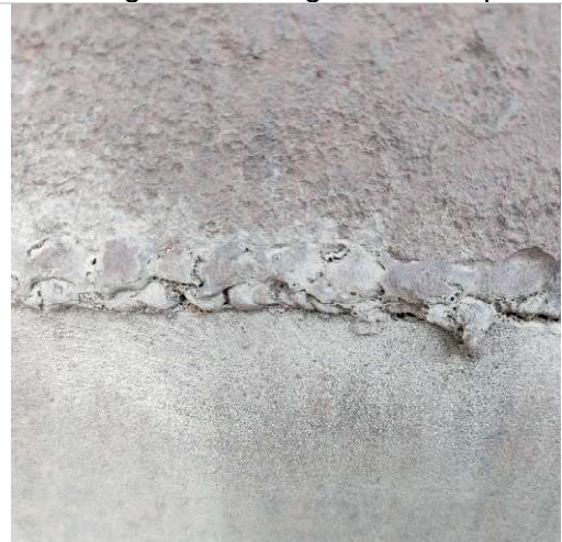
Welded splice connection between top and bottom wall sections
