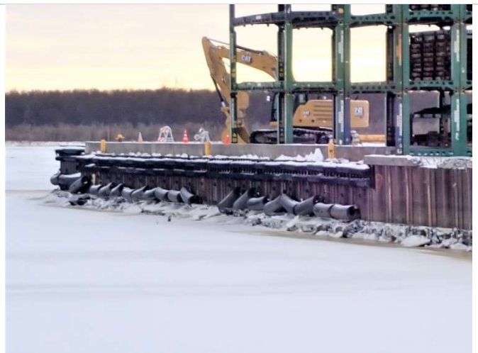
Fendering on east sheet pile wall
