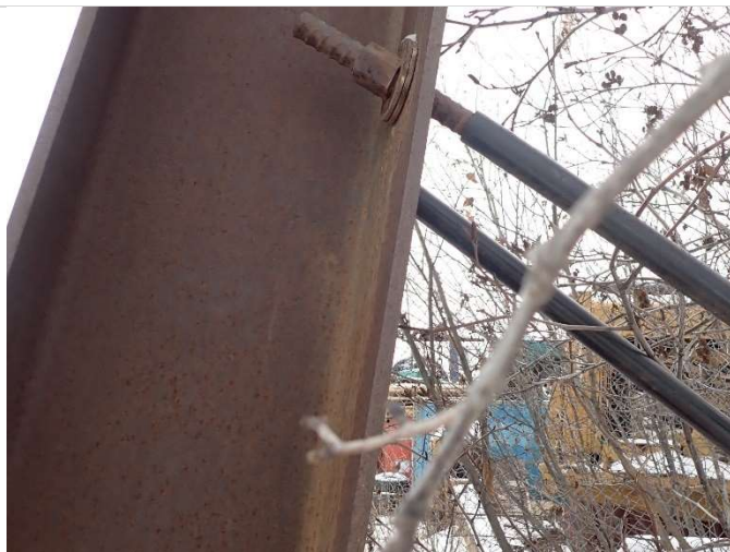
Intact HP tiebacks
