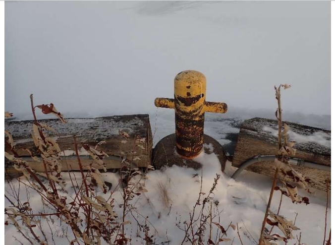
8" dia mooring bollard at intersection of east timber and sheet pile wall
