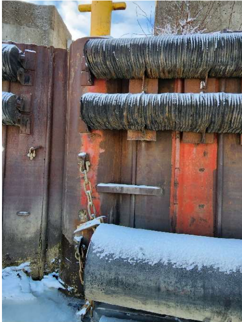
Safety ladder at soldier pile S46
