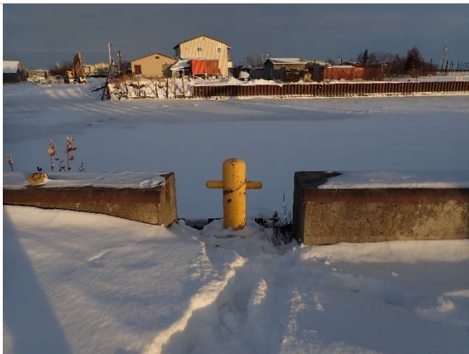
8" dia mooring bollard between concrete curbs on the east sheet pile wall.
