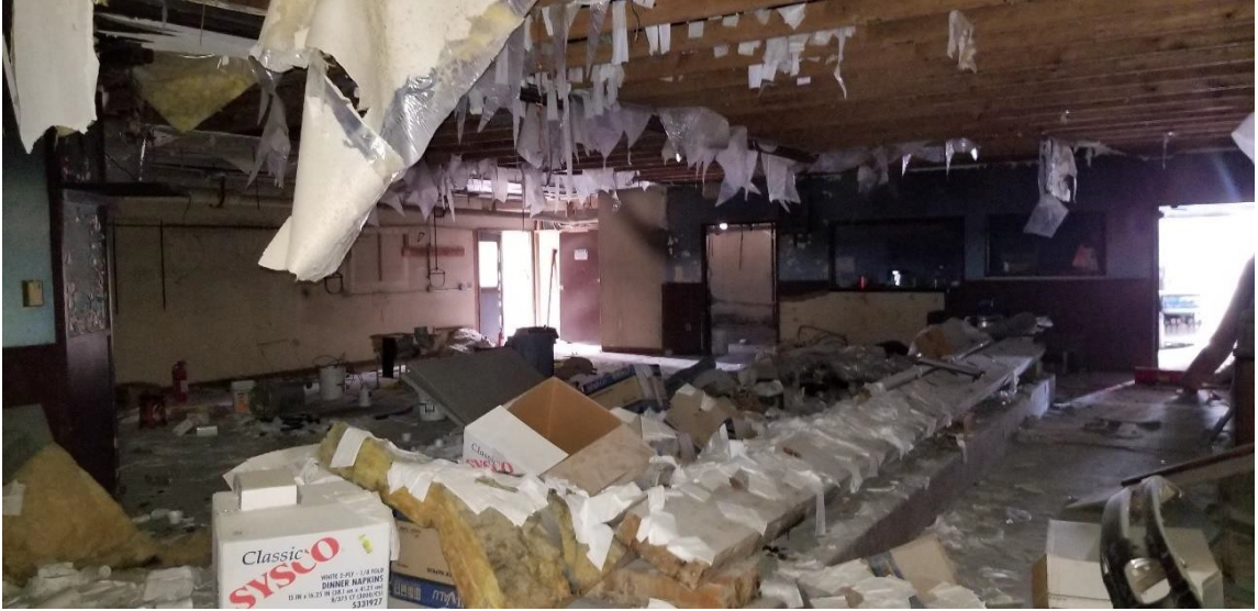
Photo 3: This photo shows the interior of the laundromat. All materials sampled tested negative for lead and asbestos.
