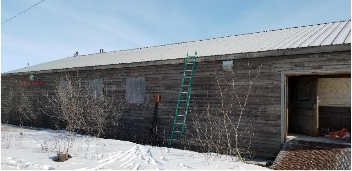
Photo 1: This photo shows the exterior of the laundromat. The roof consists of corrugated metal overtop felt paper and the exterior wall consist of wood clapboard overtop wood panel.
