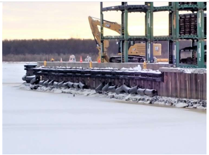
Fendering on east sheet pile wall
