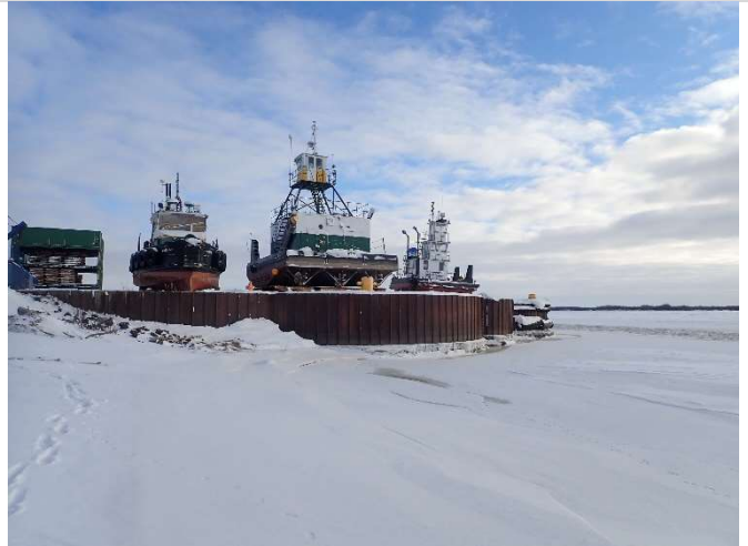
Elevation view of the west wing wall and armour rock protecting the wall's shoreward toe
