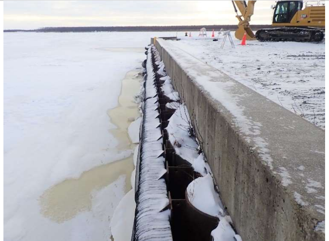
Concrete curb and fendering along east sheet pile wall
