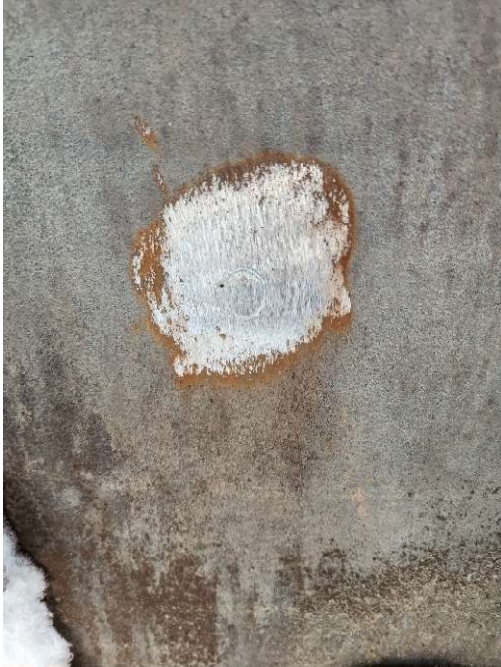
Prep area for UT thickness remaining measurement
