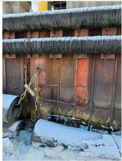
Safety ladder at soldier pile S37
