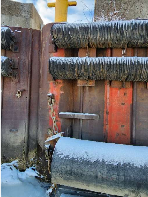
Safety ladder at soldier pile S46
