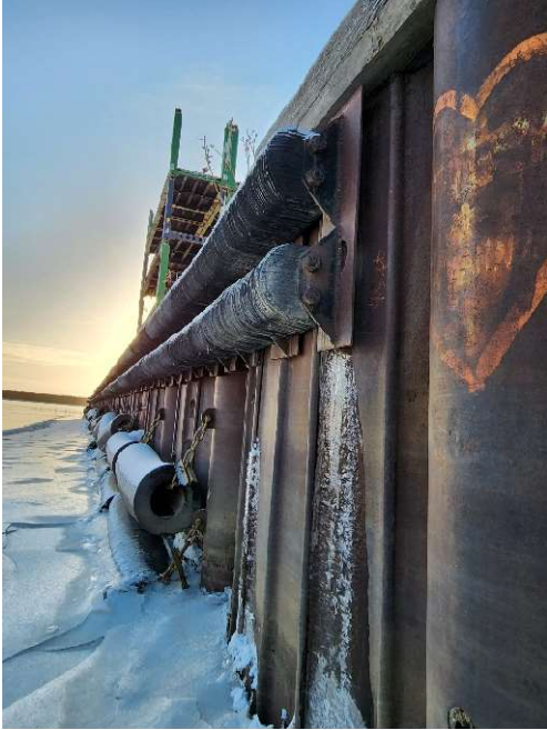
Start of east wall fendering
