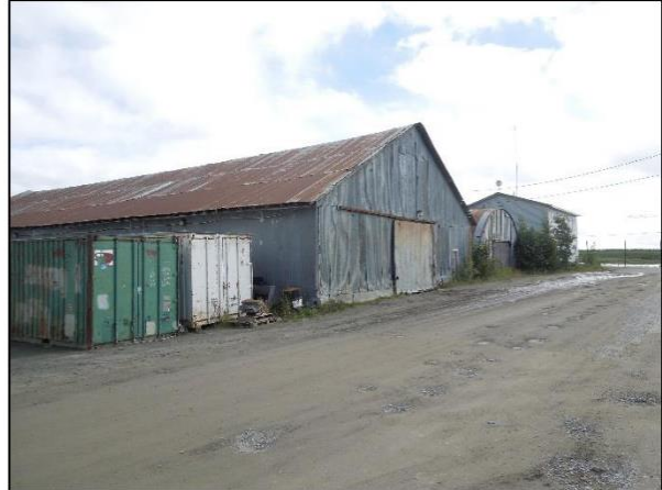
Warehouse, Main St looking south
