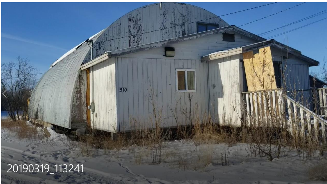
Photo 1: This photo shows the former Bethel police barracks. None of the exterior materials tested positive for lead based paint or asbestos.
