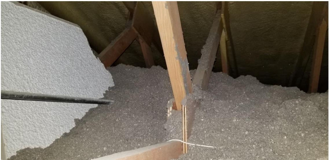
Photo 4: This photo shows the attic insulation present in select areas of the building. This material was also negative for asbestos.
