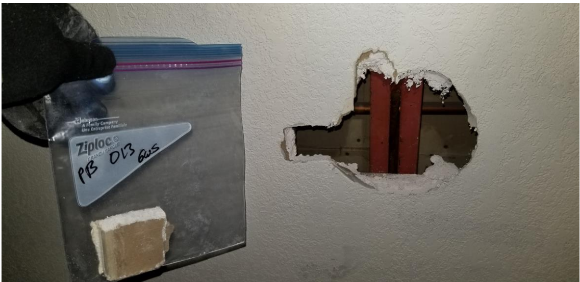
Photo 6: This photo shows one of the many samples of wall textures collected. All wall textures were found to be non-ACM. This photo also shows where the wall was opened to look for hidden materials, such as pipe insulation.
