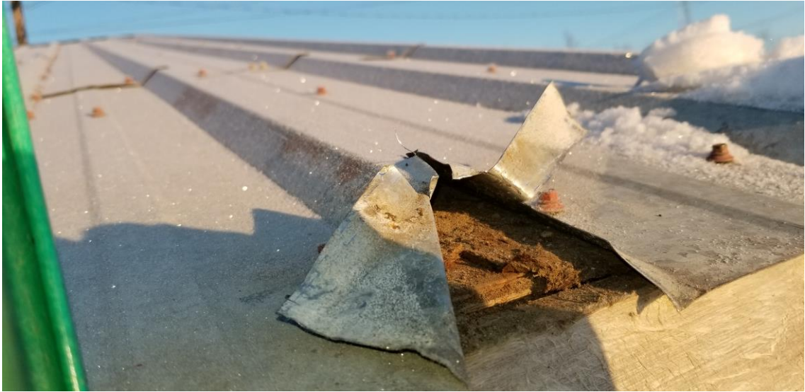
Photo 3: This photo shows the roof materials present above the entryway. All roof products tested were negative for asbestos.
