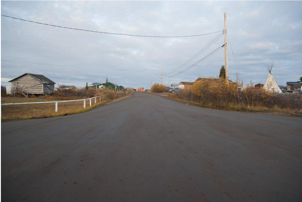
Hard smooth gravel road surface treated with EK35
