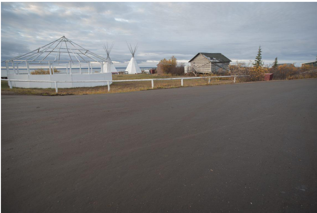
Pavement like EK35 road surface
