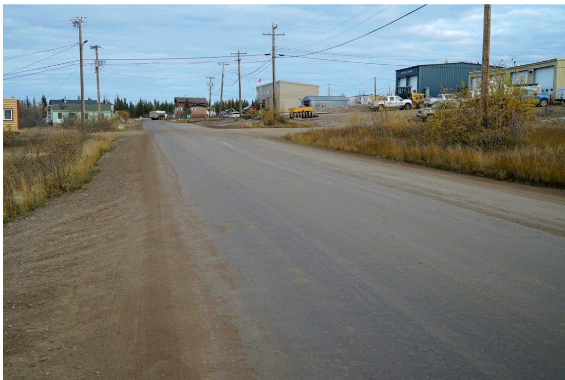
Tightly bound treated road surface
