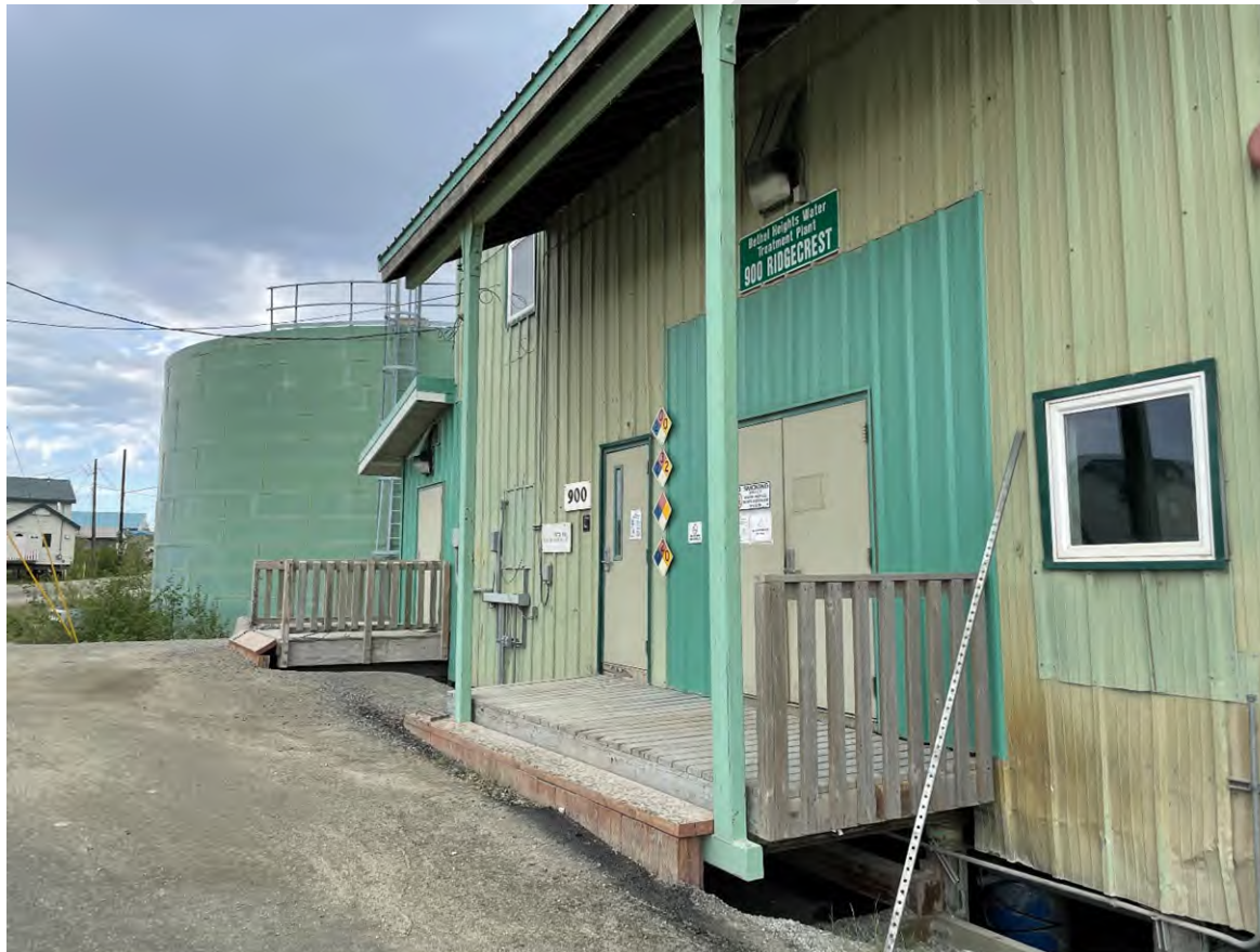
Bethel Heights water treatment plant.
