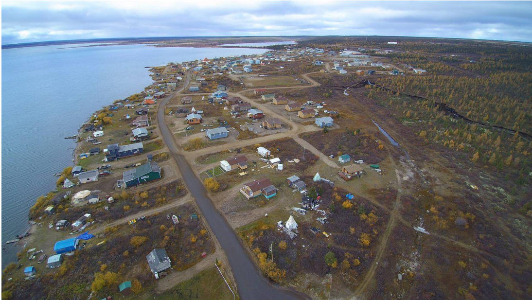
Aerial view of Delani NWT Road treatment
