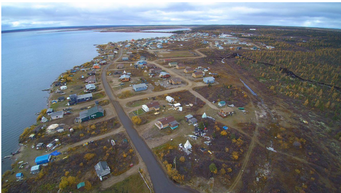
Aerial view of Delani NWT Road treatment
