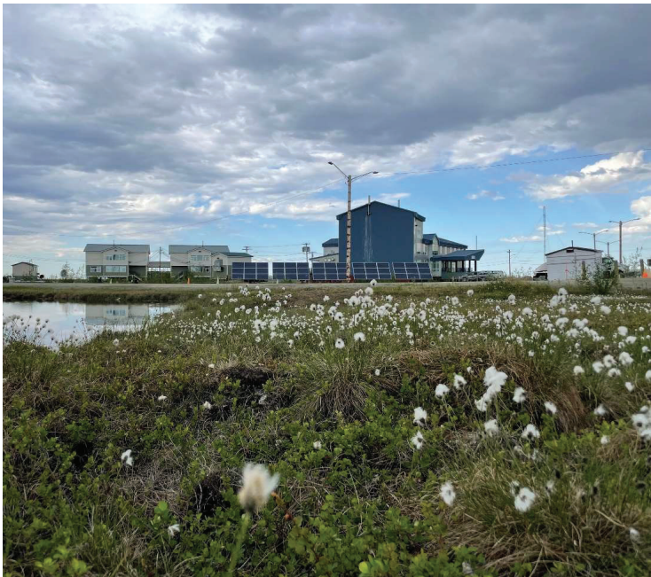
A solar array near the Fitness Center in Bethel.
