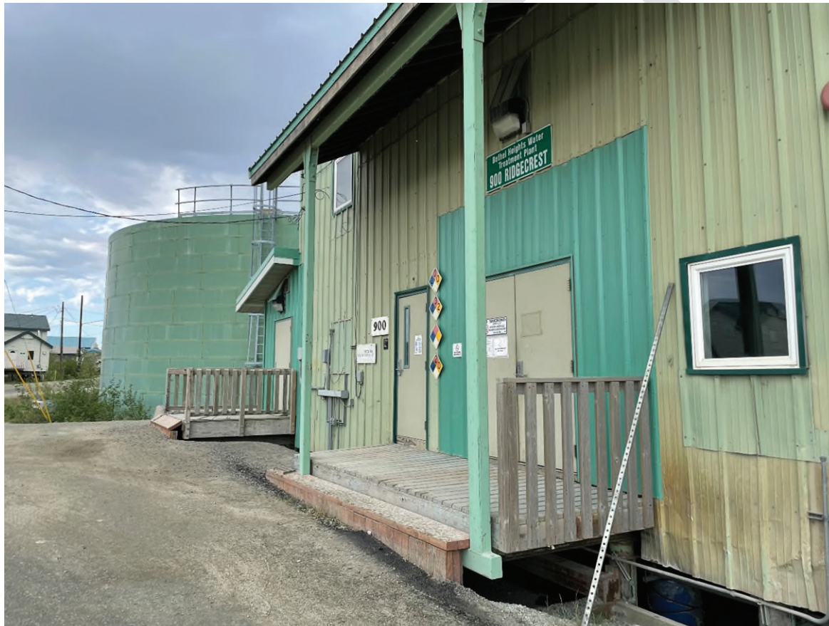
Bethel Heights water treatment plant.
